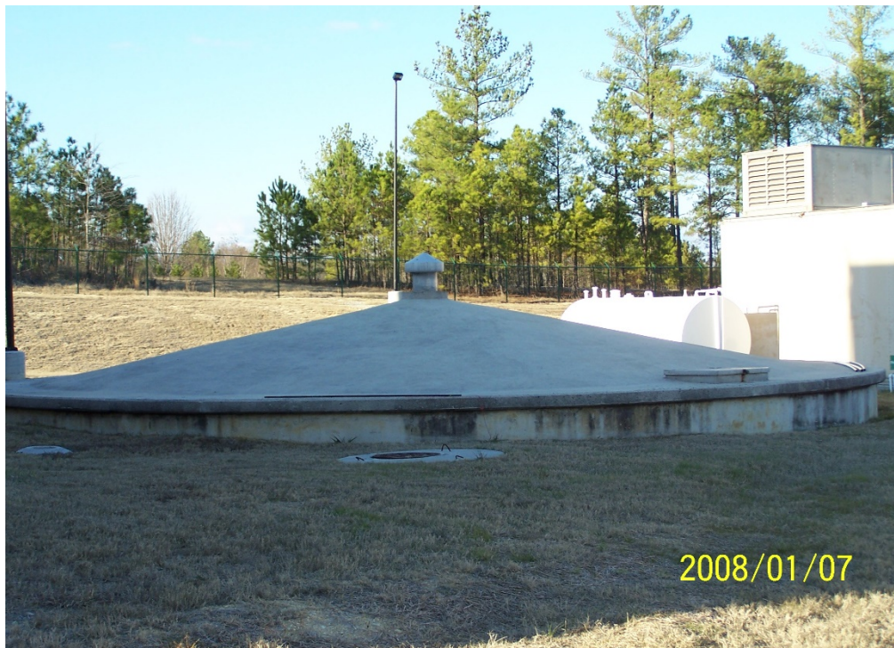
The older clearwell holds 100,000 gallons of finished water
