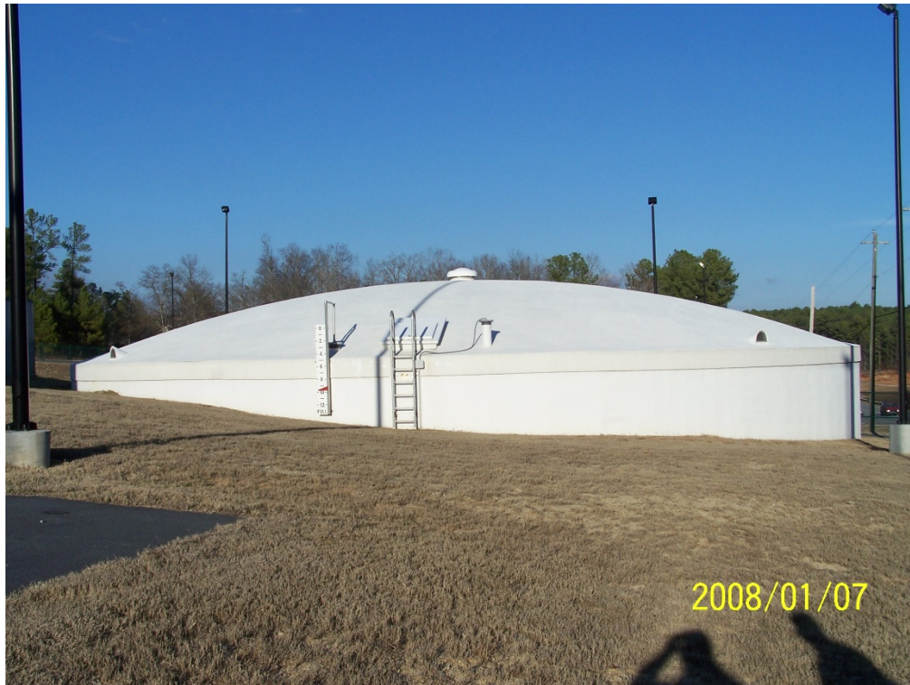
The newer clearwell holds 500,000 gallons of finished water
